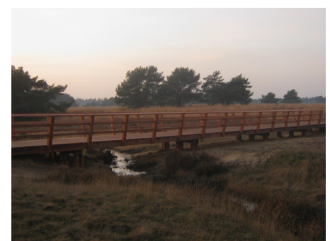
Deelense Veld – new bridge and creek
