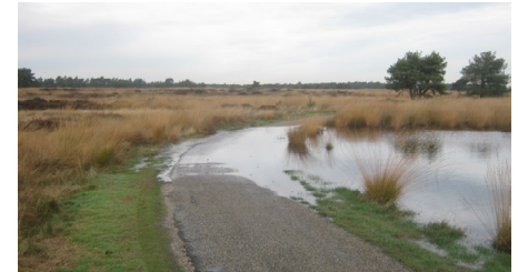
problems with the cycling path
