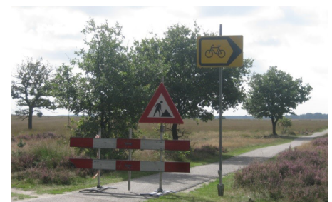
Signing during construction
